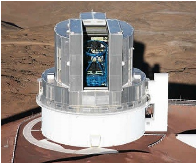
Subaru Teleskope from: https://www.nao.ac.jp/en/project/hawaii.html
